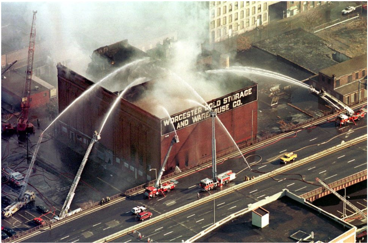
Figure 1.1: A photo of a severe structural fire that occurred on December 3 1999 in Worcester, Massachusetts [52].
