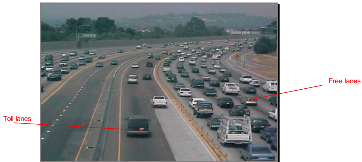
Figure 2. New lanes on SR-91
