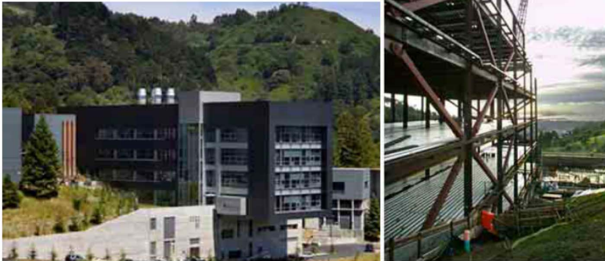
Figure 4. Experimental test site. Left: the Molecular Foundry building at LBNL. Right: view of the building during construction revealing the steel decks between floors.
