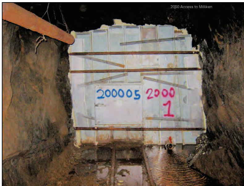
Figure 5.4.3.8.1-2 Kennedy Stopping on the 2000L. [SDSTA]
