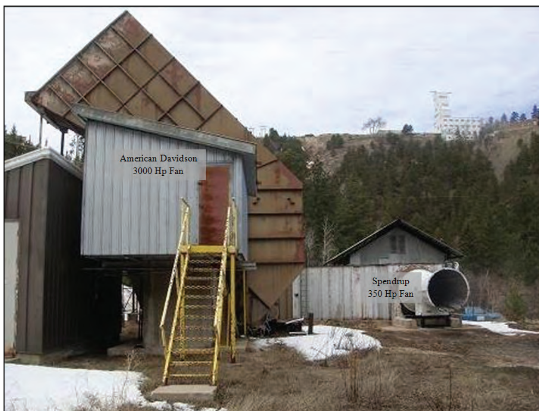
Figure 5.4.3.8.1-3 Oro Hondo Shaft current configuration. [SDSTA]
