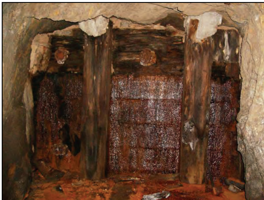
Figure 5.4.3.12.1-4 Leaking former Homestake mine stope wall on the 2000L. [SDSTA]
