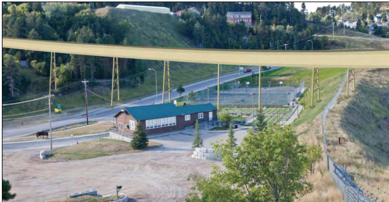
Figure 5.4.3.9.4-5 Depiction of what the pipe conveyor will look like to the community. [SRK]
