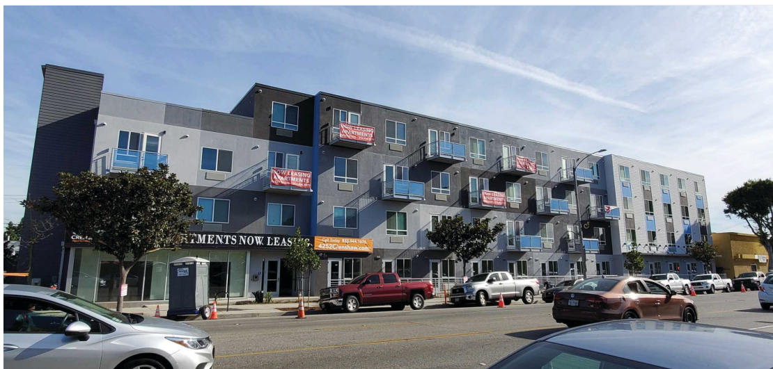
A parking-free 111-unit modular housing development at 4252 Crenshaw Blvd. Source: Urbanize LA.
