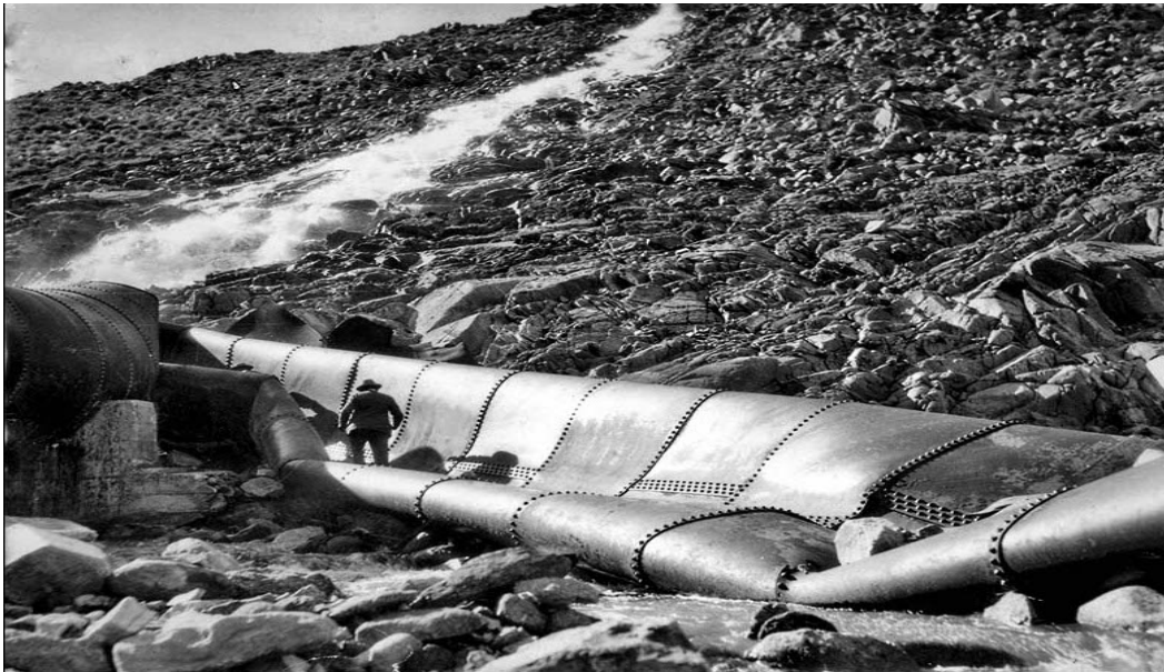
Water gushing from the Aqueduct after protestors use dynamite in 1927. 7
