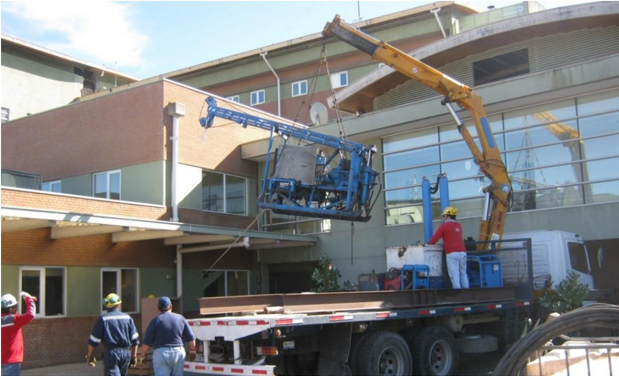
**Fig. 4.6.** Lowering SPT equipment into position
