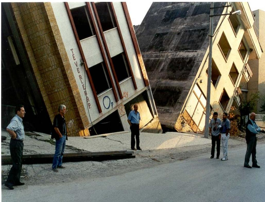
**Fig. 3.1.** Two adjacent buildings that tilted away from each other due to liquefaction in foundation soils (Bray et al. 2000)
