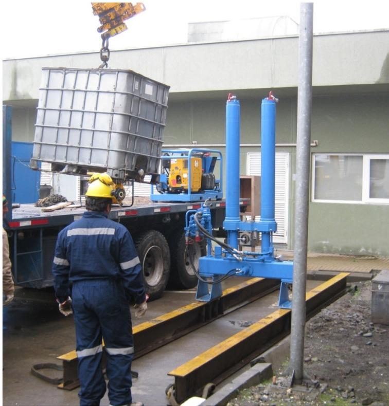
**Fig. 4.2.** CPT frame in position with a concrete counterweight being placed
