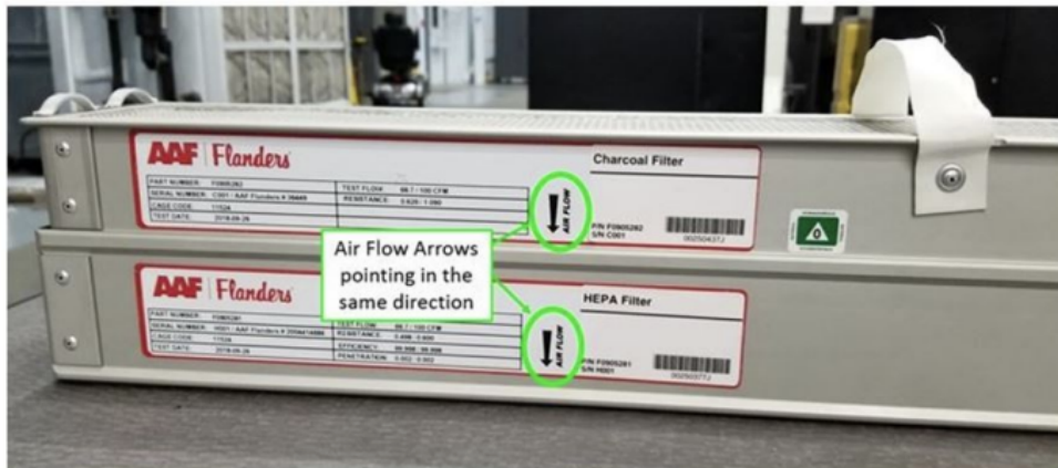
Figure 13. Airflow Arrows on Charcoal and HEPA Filters.
