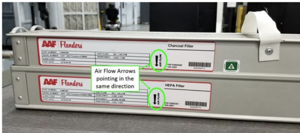
Figure 8. Airflow Arrows on Charcoal and HEPA Filters.
