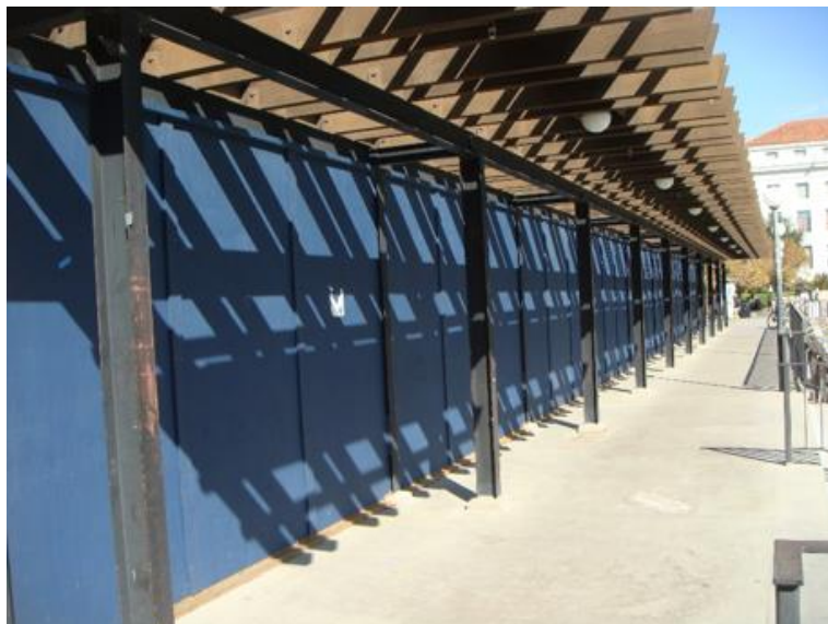
Figure 1.2-15: Windows blocked with plywood for acoustical mitigation of construction noise
