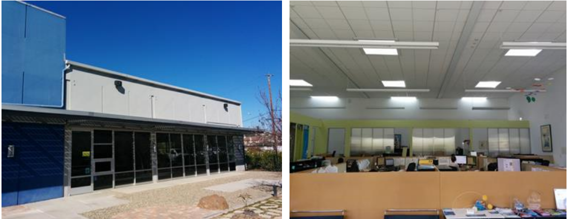
Figure 1.4-1: IDeAS building exterior, left, and interior, right
