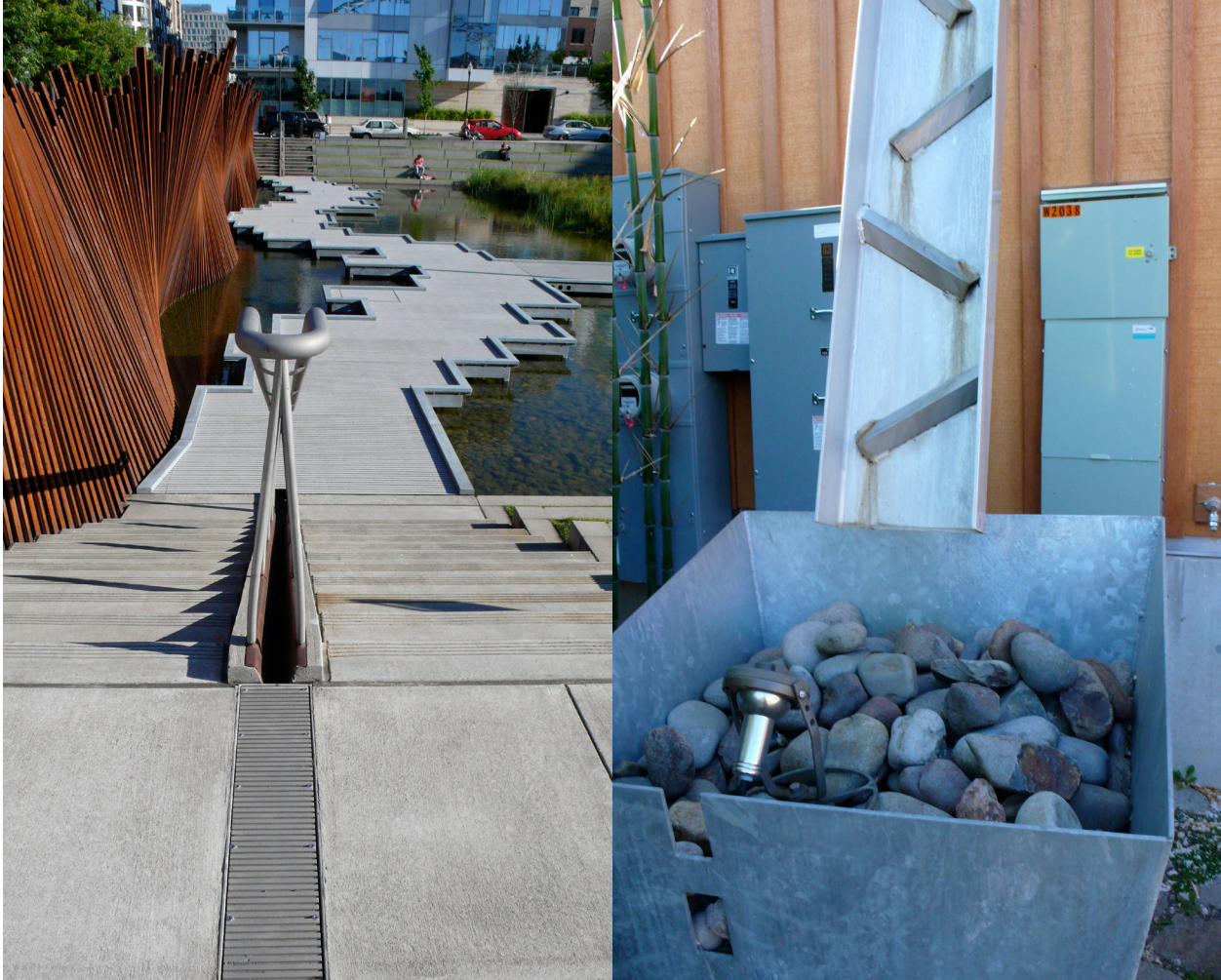
Figures 14 and 15 Left: A trench drain and runnel along a staircase in Portland, Oregon. Right: an energy dissipation bucket that overflows to a runnel. (photos by Andrea Gaffney)
