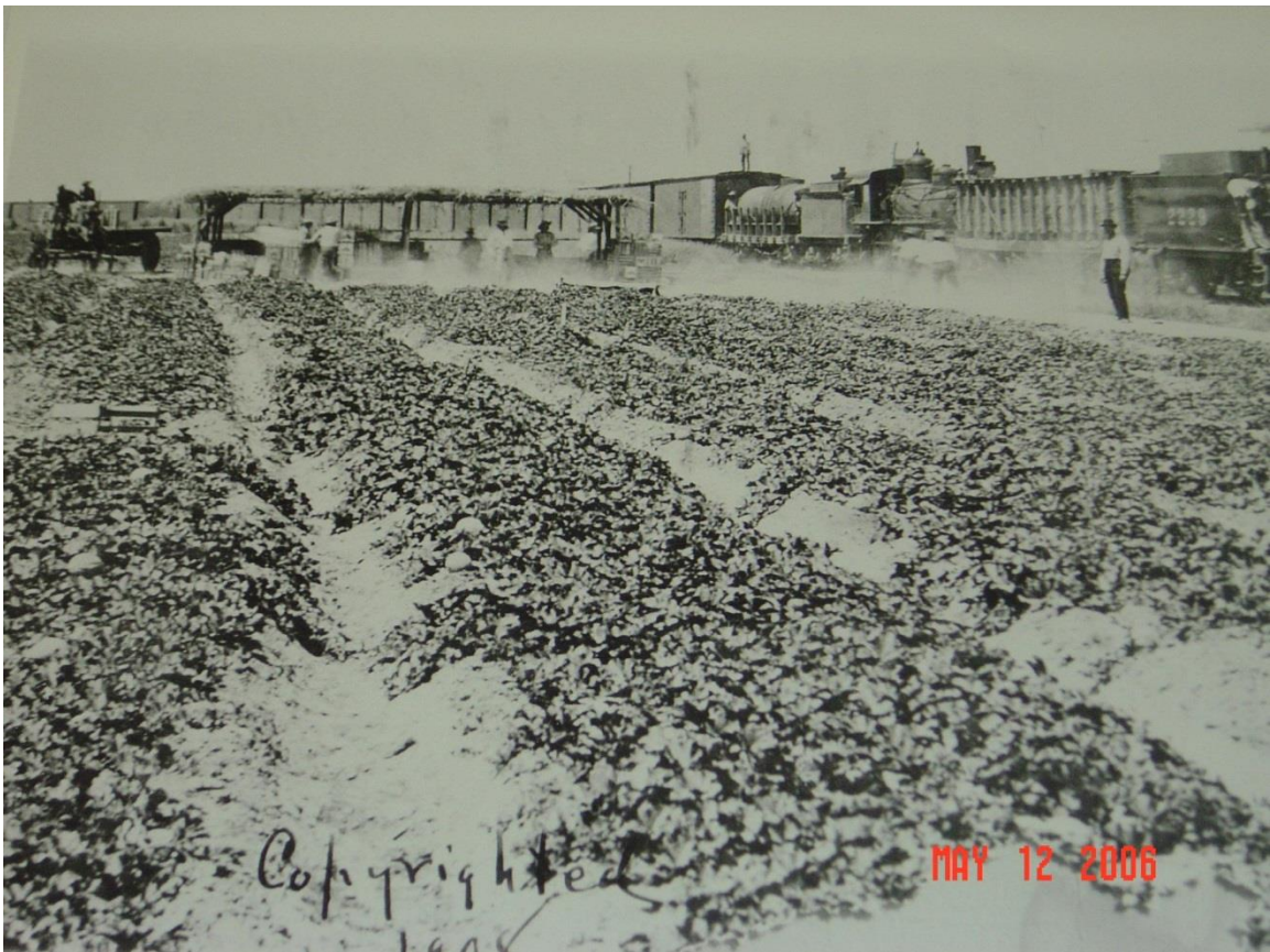
Figure 3 – Loading Produce Directly to Rail Cars in 1908
