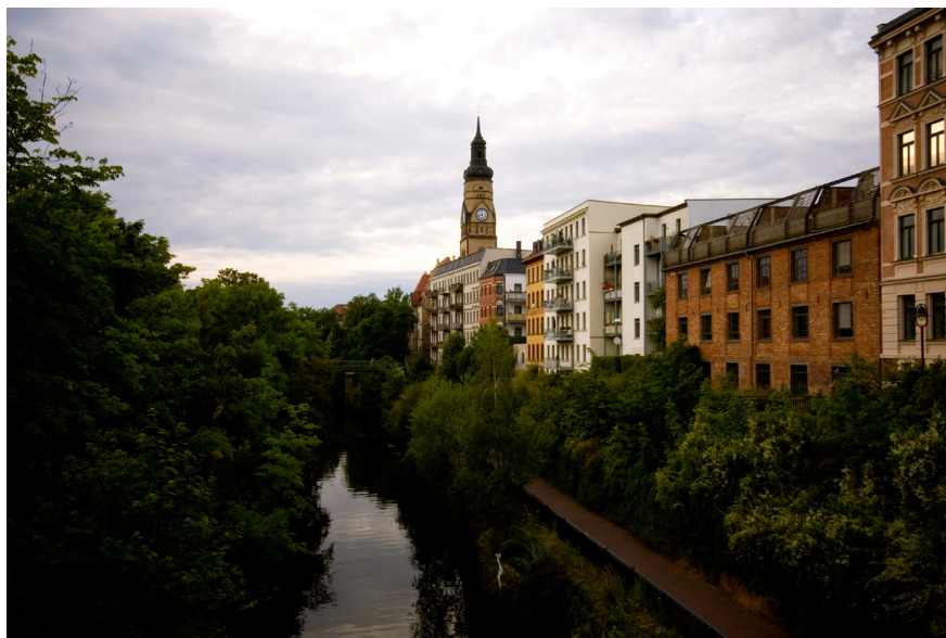
Figure 7. New residential development along Karl-Heine-Kanal.
