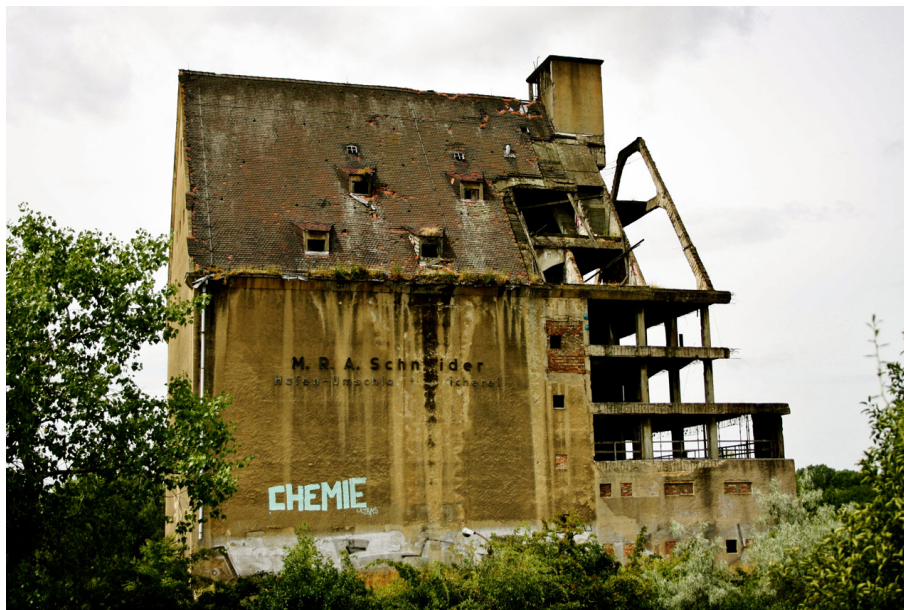
Figure 2. After reunification, Leipzig lost more than 75% of local industry, leaving behind many abandoned industrial buildings such as this former grain refinery.
