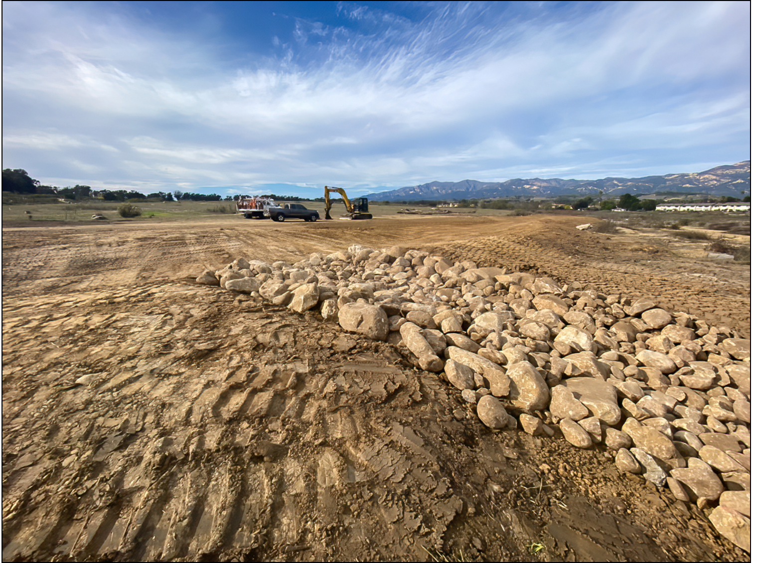
This overflow channel will direct water towards the remnant willow patch.
