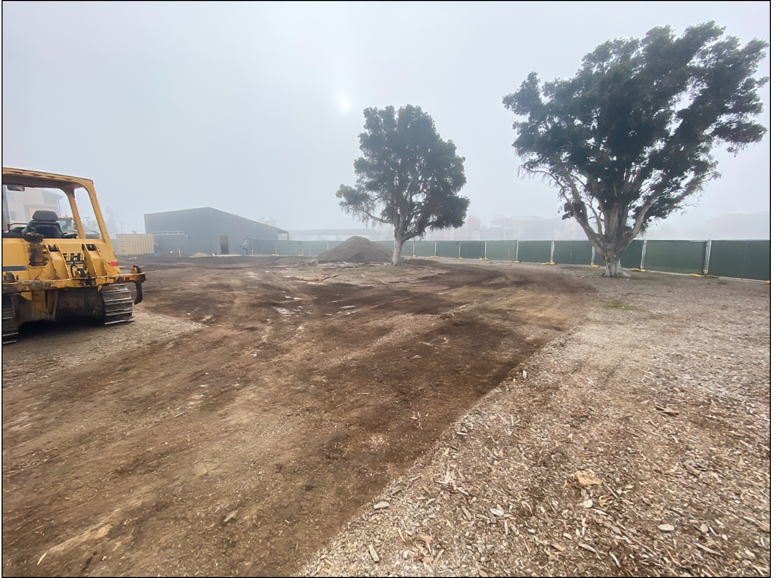
Grading for outdoor classroom.
