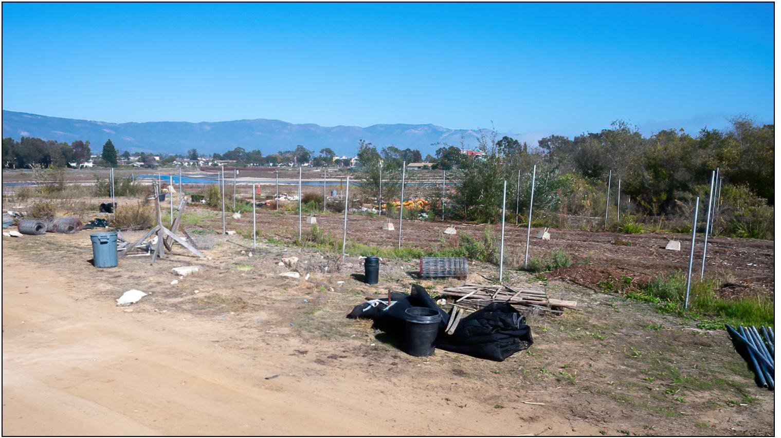
Removal of the shade-structure.
