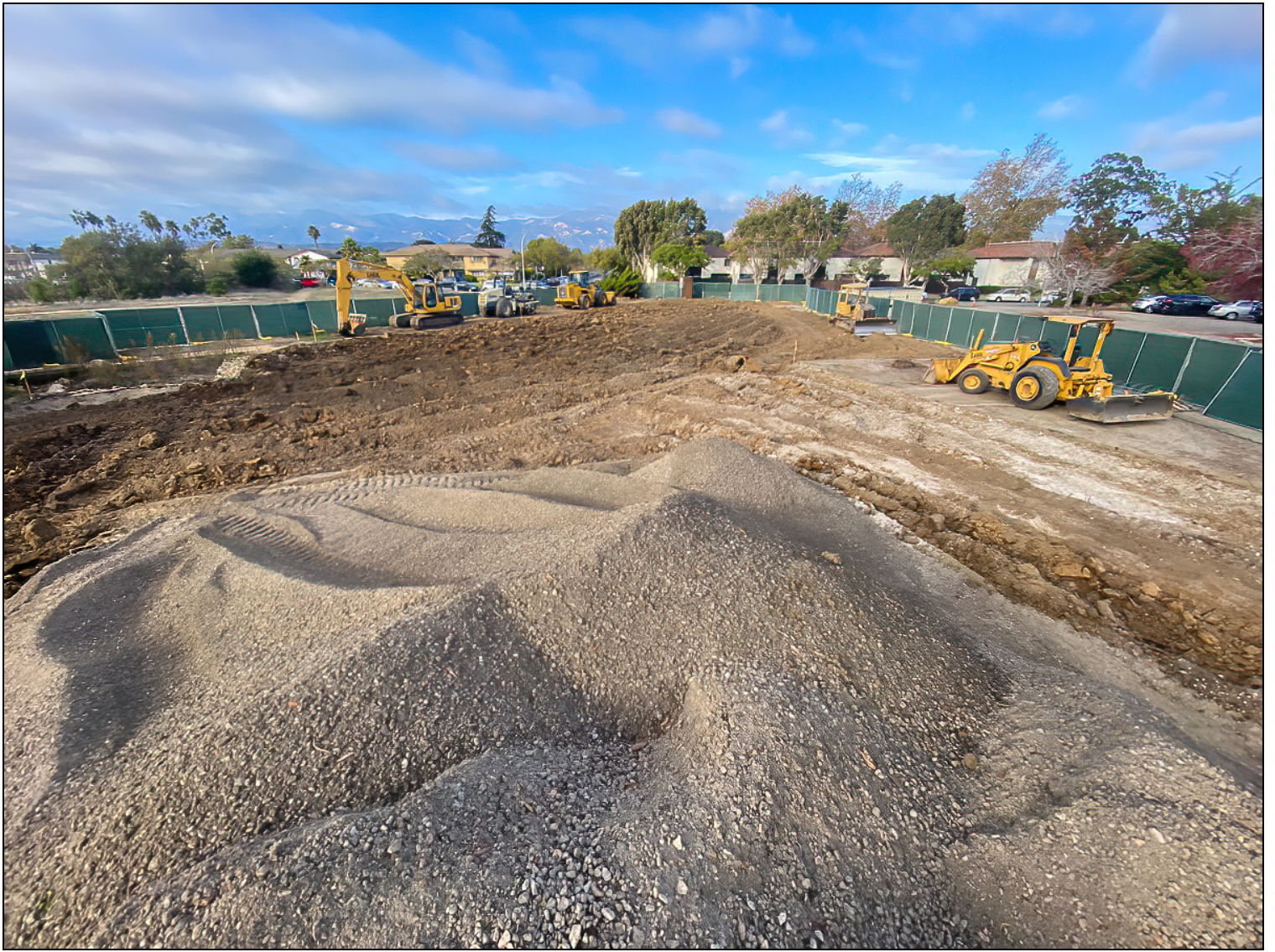
Removal of the old parking lot.
