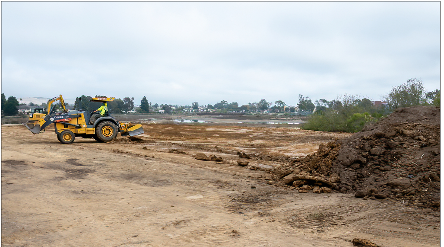
Dense clay soils require heavy equipment to reshape.
