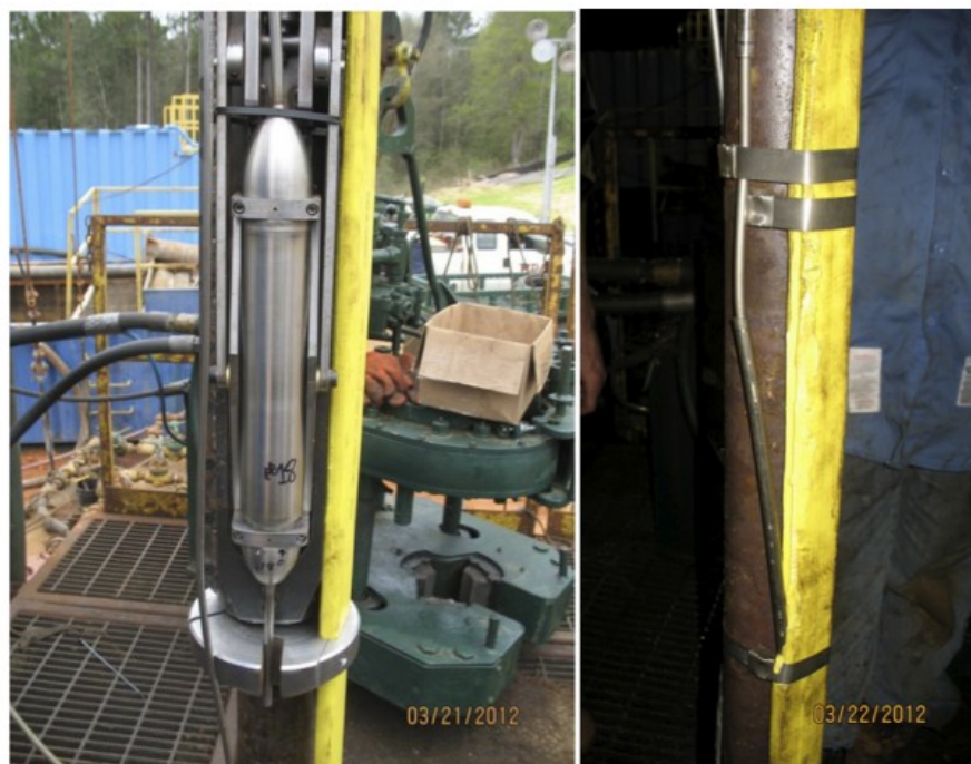
Figure 4 (left) MBM geophone with a hydraulic clamp, mounted on tubing with yellow flatpack. (right) Flatpack with a hydraulic line, each attached to tubing with steel banding. The DAS data were recorded using a fibre inside the flatpack, clamped to tubing as shown with clamps every \sim 10 m and banding every \sim 5 m.
