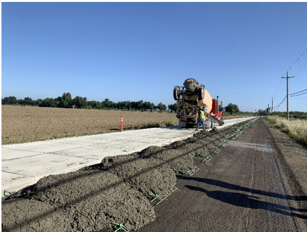
Asphalt surface is adequately wet conditioned: uniformly moist but free of standing or flowing water
