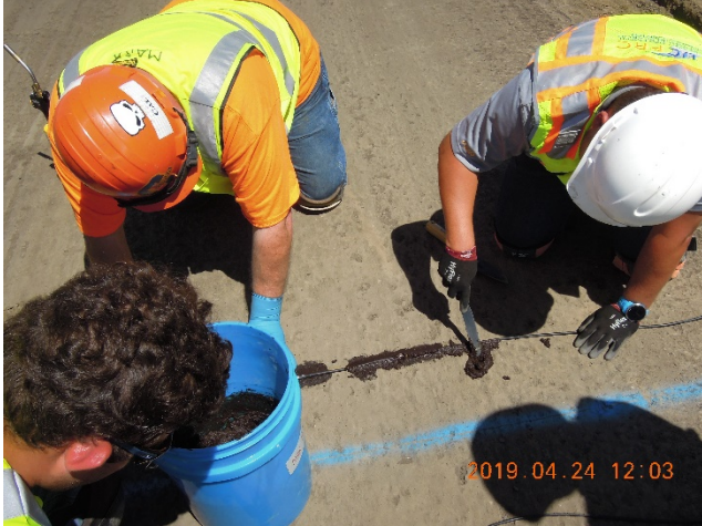
Fixing strain gauge cable with sand-cold mix asphalt
