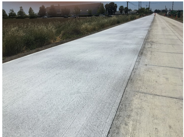
Appearance of the final surface
