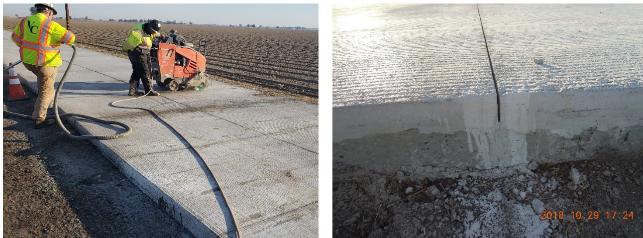
Figure 4.28: Sawcutting operation.
