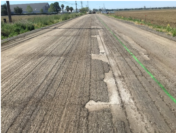
Segment A: Asphalt cracking and areas with delamination
