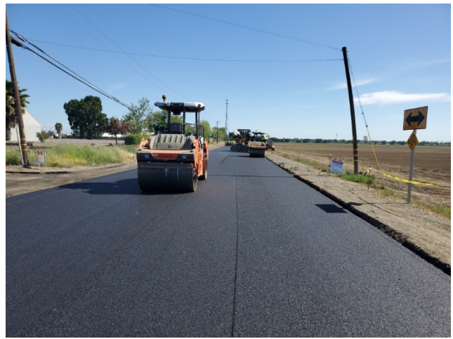
Figure 4.9: Asphalt placement and compaction.
