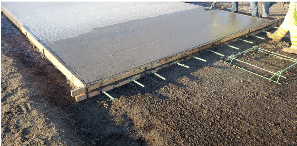
Figure 4.24: Installation of tie bars instead of dowels at a transverse joint (end of paving Shift 1).
