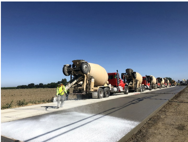
Manual spraying of curing compound
