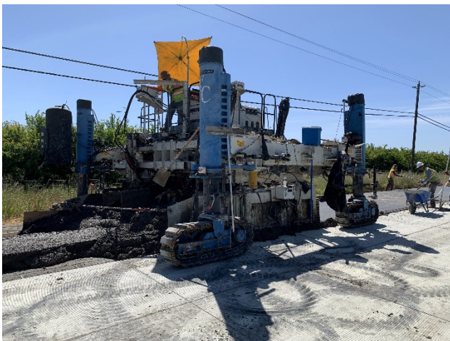
Figure 4.20: Slipform paver.
