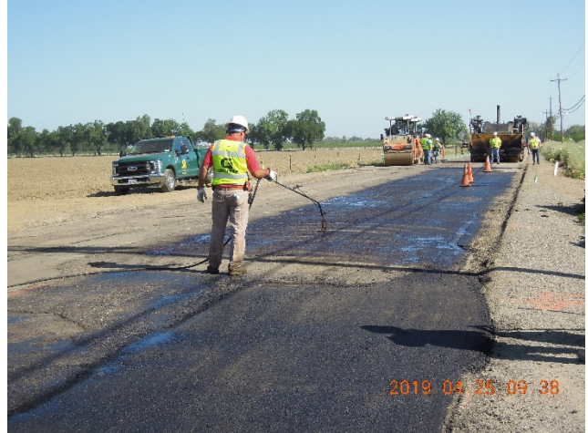
Tack coat application
