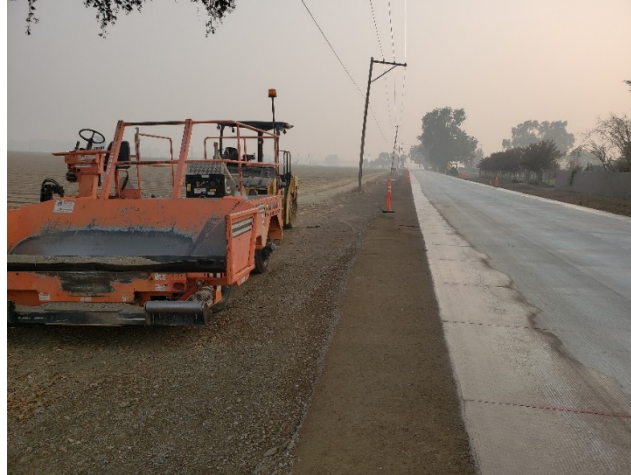
Figure 4.29: Shoulder backfilling.
