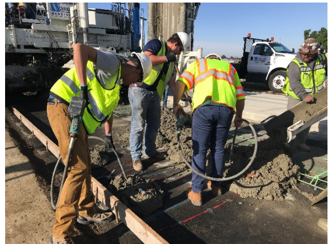
Consolidating the concrete around the sensors
