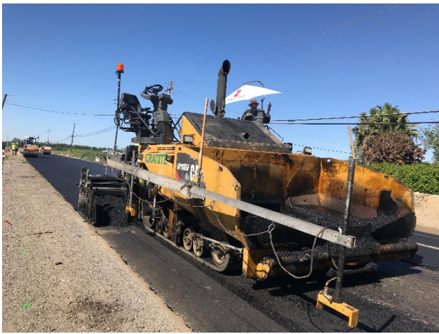
Figure 4.9: Asphalt placement and compaction.
