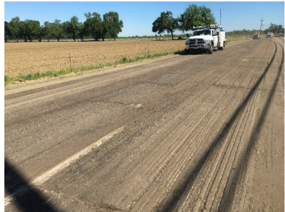
Segment A: Asphalt cracking and areas with delamination
