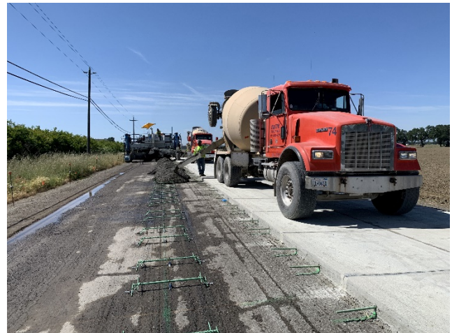
Asphalt surface is not adequately wet conditioned: some dry areas; standing water at the shoulder
