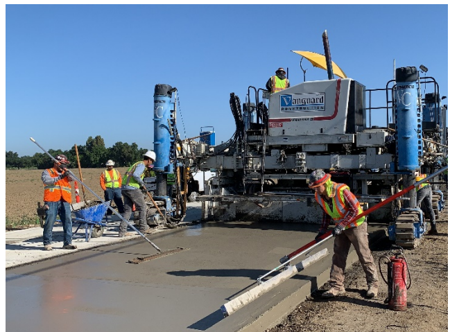
Figure 4.20: Slipform paver.
