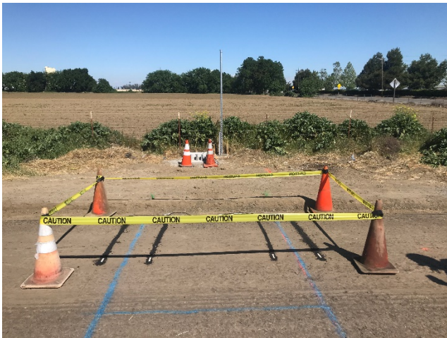
Strain gauge and cable protection until RHMA-G placement
