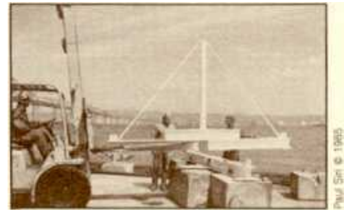
BML personnel attach a mooring superstructure to concrete blocks.
