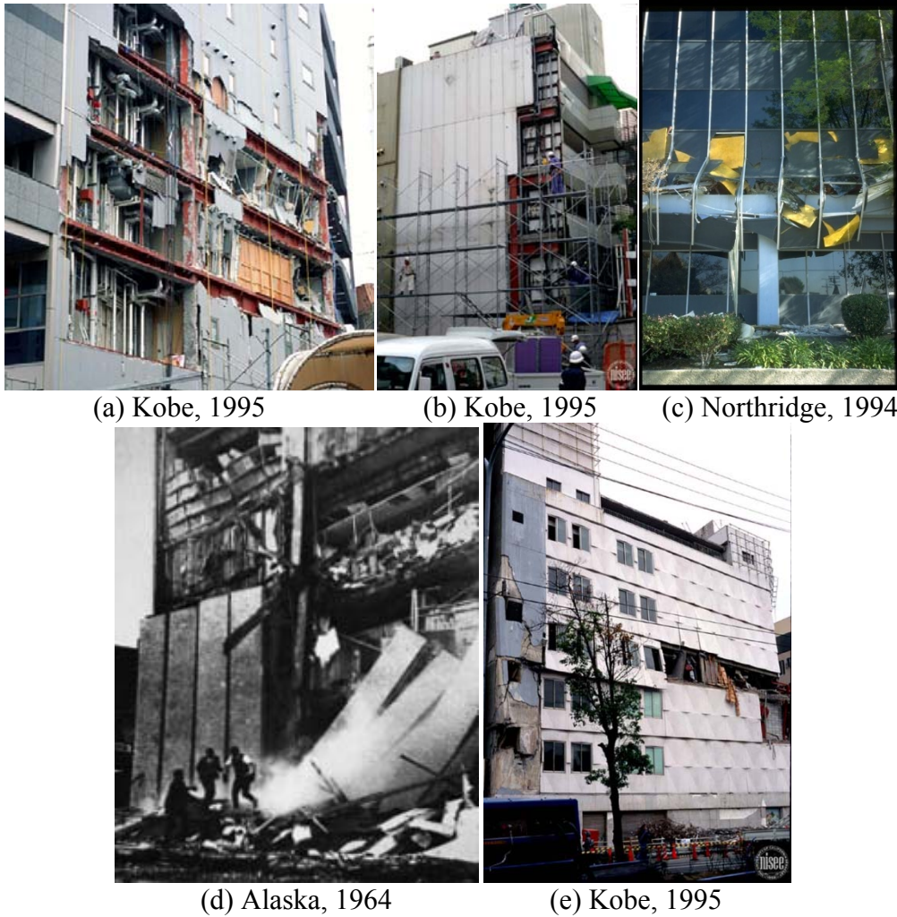
Fig. 1.21 Photographs of cladding damage in past earthquakes (PEER Library)
