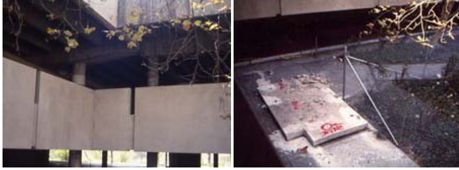
Fig. 1.22 Parking structure at California State University, Whittier earthquake 1987: left, cladding panels; right, fallen concrete panel, causing fatality (Arnold, 2008).
