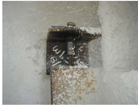
Vertical bearing connection
