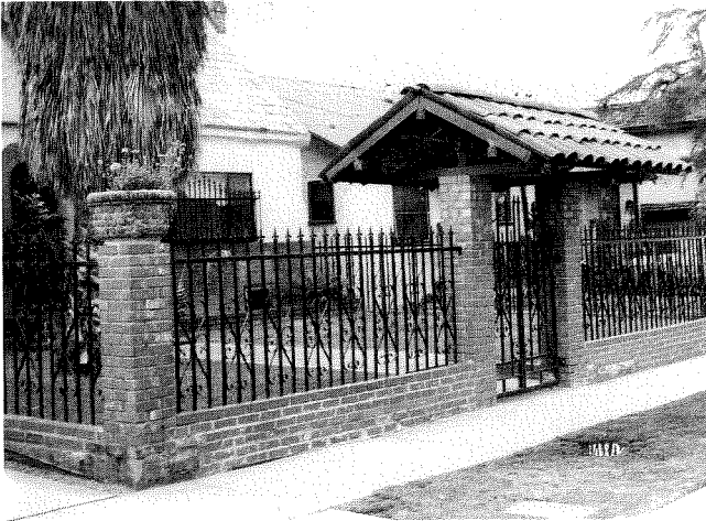
Fences and thresholds help extend household space to the street.
