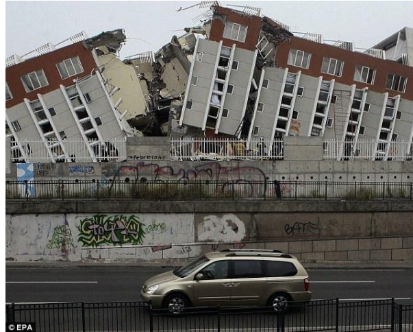
(d) Apartment building seriously damaged by 1994 Northridge earthquake.
