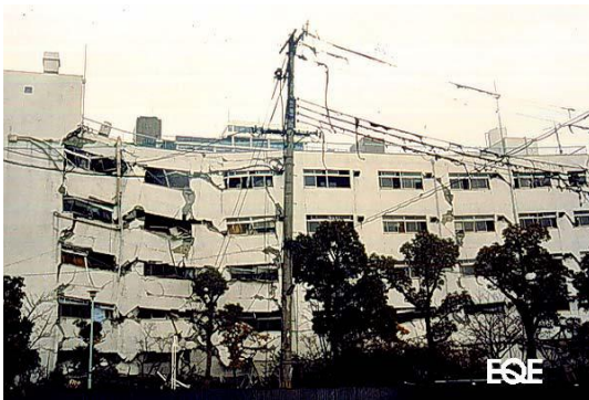
(b) Kobe earthquake damage. Failure of the first story caused partial collapse of upper stories.
