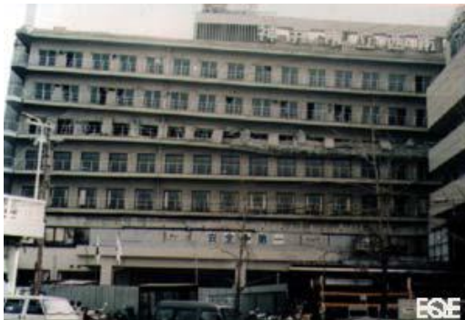
(b) Kobe earthquake damage. Failure of the first story caused partial collapse of upper stories.
