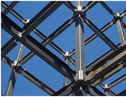
(a) steel moment frame inner-view
