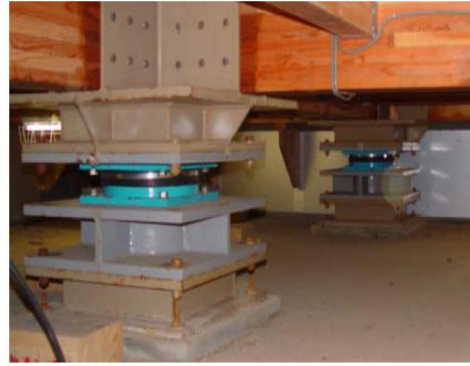
(b) FPS system construction
