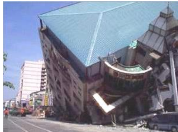
(e) A collapsed building located in Nantou County from 1999 Jiji earthquake.
