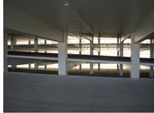
(b) Inside view of parking building
