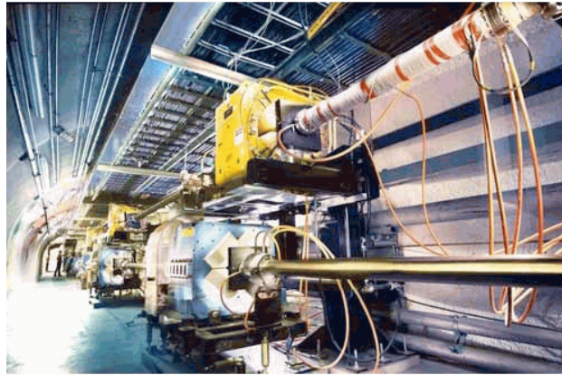
Figure 1 View of the PEP-II tunnel.
