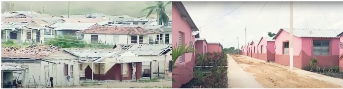
Figure 4. 11: The houses of Emilio Cordoba before and after the hurricane
