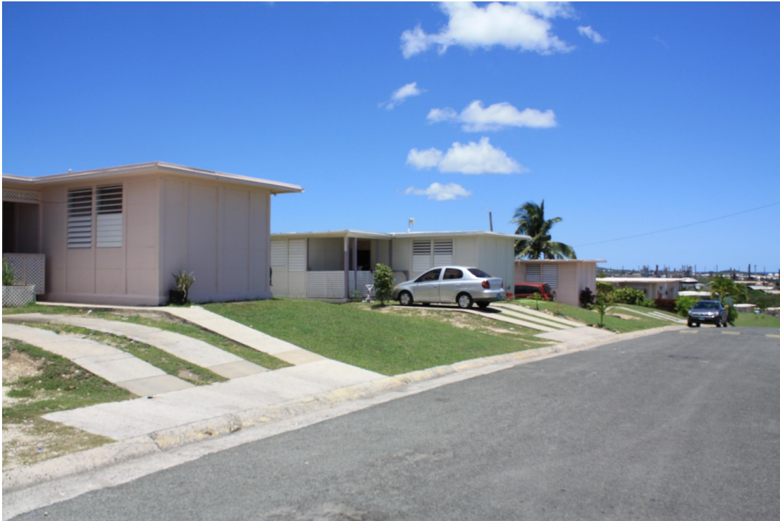
Figure H: Ms. Hanks’s neighborhood. In the background in the far right, you can see the towers of the defunct aluminum plant whose employees these homes were originally meant to house.
