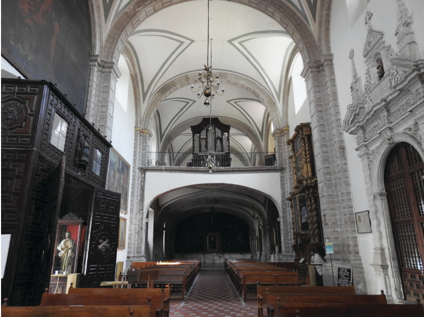
Figure 2.4 Coros with modified coro bajo to lengthen nave, Regina Coeli convent, Mexico City, built ca. 1732
