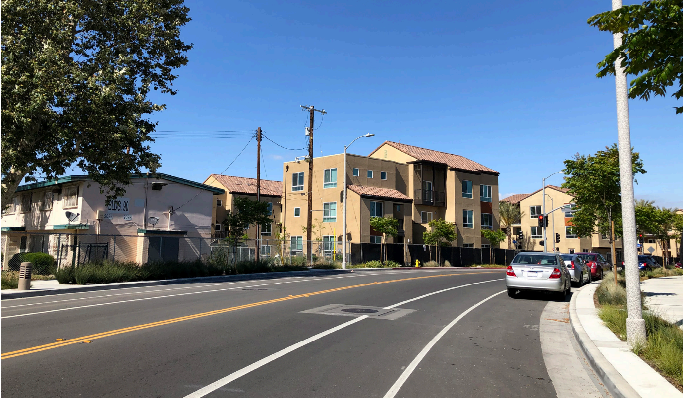
New bicycle lanes on Century Blvd. Site of new Jordan Downs development.
