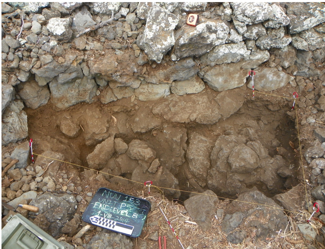
Figure 7.5: The foundation of the NUU-153 Units P5 and P6 east wall showing the bedrock foundation.
