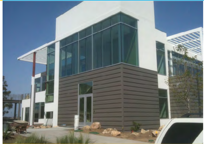
West facade of the new modular office on the Long Beach Gas and Oil campus
