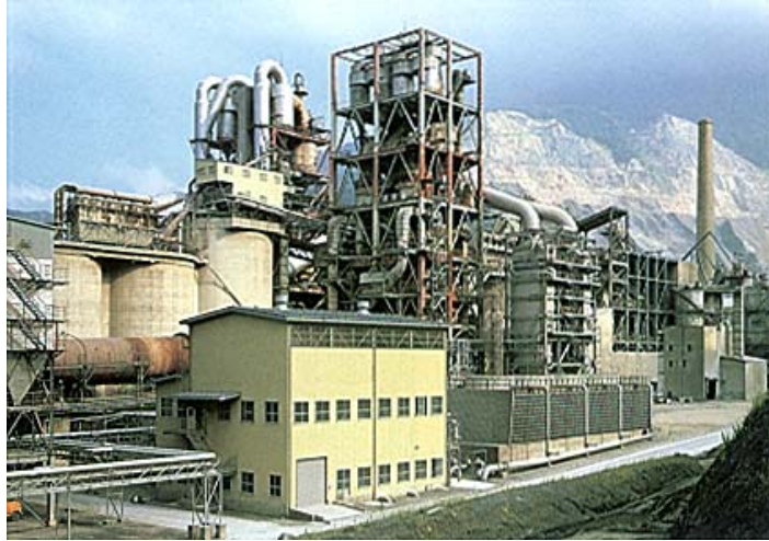
Waste heat recovery at cement plant, image taken from http://www.takuma.co.jp/english/product/boiler/hainetu/cement.html
