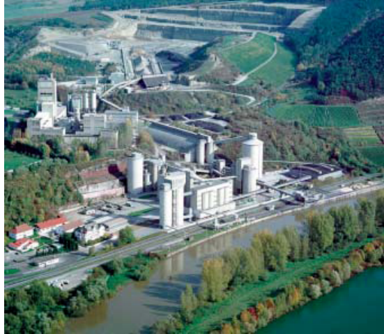
1.5 MW Ormat ® Energy Converter at the Lengfurt Cement, Germany, image taken from http://www.ormat.com/FileServer/70b593358e2da845c512c50dc0c47613.pdf
