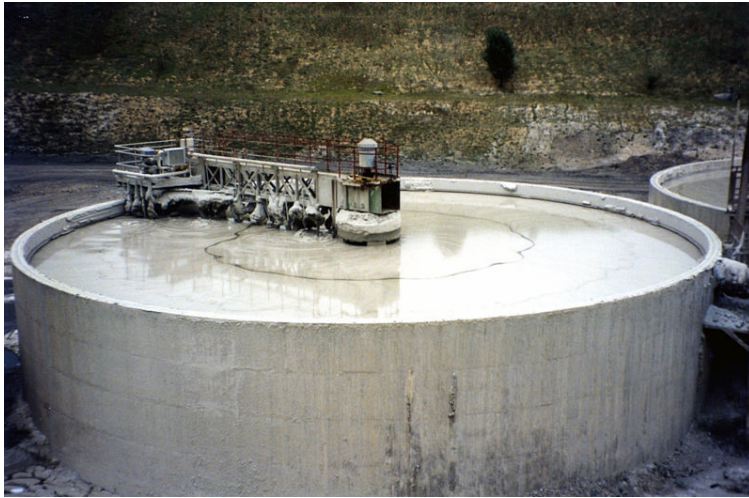
Slurry storage and blending tank, image taken from Wikipedia, http://en.wikipedia.org/wiki/Rawmill
