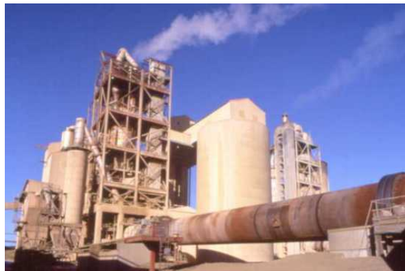
View of a cement kiln and preheater tower. Picture courtesy Castle Cement, at http://www.understanding-cement.com/manufacturing.html
