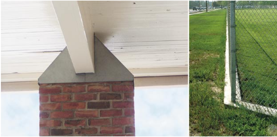
Less-toxic practices to prevent school pests include: left , designing buildings to prevent roosting pigeons, which can carry diseases, and, right , installing mowing strips to prevent weed growth along fence lines.
