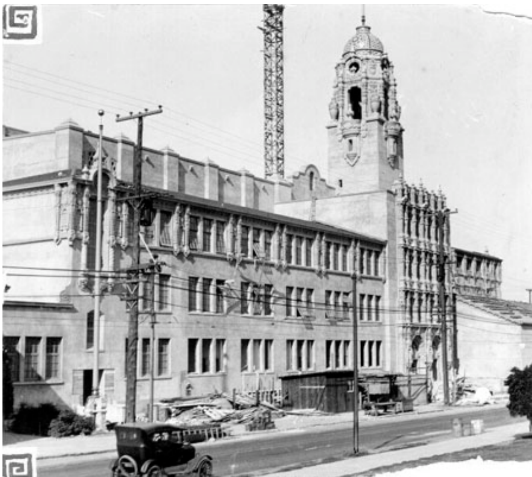
Figure 17: 1926 photograph of Mission High School. Source: San Francisco Historical Photograph Collection, San Francisco Public Library, Photo ID Number: AAB-0389.
