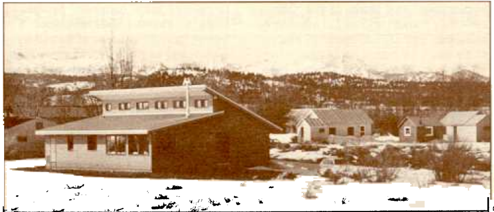
SNARL's newly completed housing facility, shown in foreground, adds living space for 28 researchers and students based at this eastern Sierra Nevada site.
