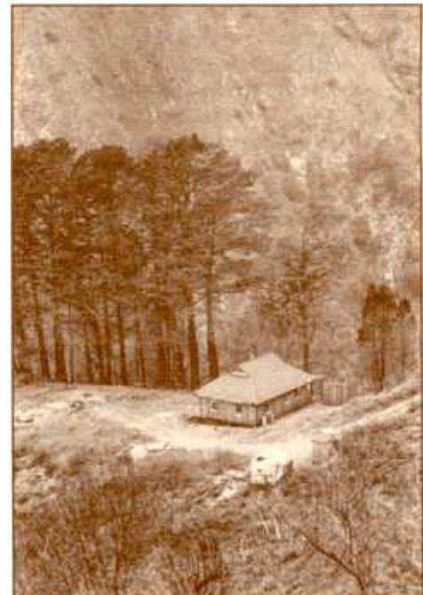
Big Creek's new steward's cabin, which sits atop a 600-foot ridge overlooking the Pacific, is one of the facilities rebuilt since the fire.
