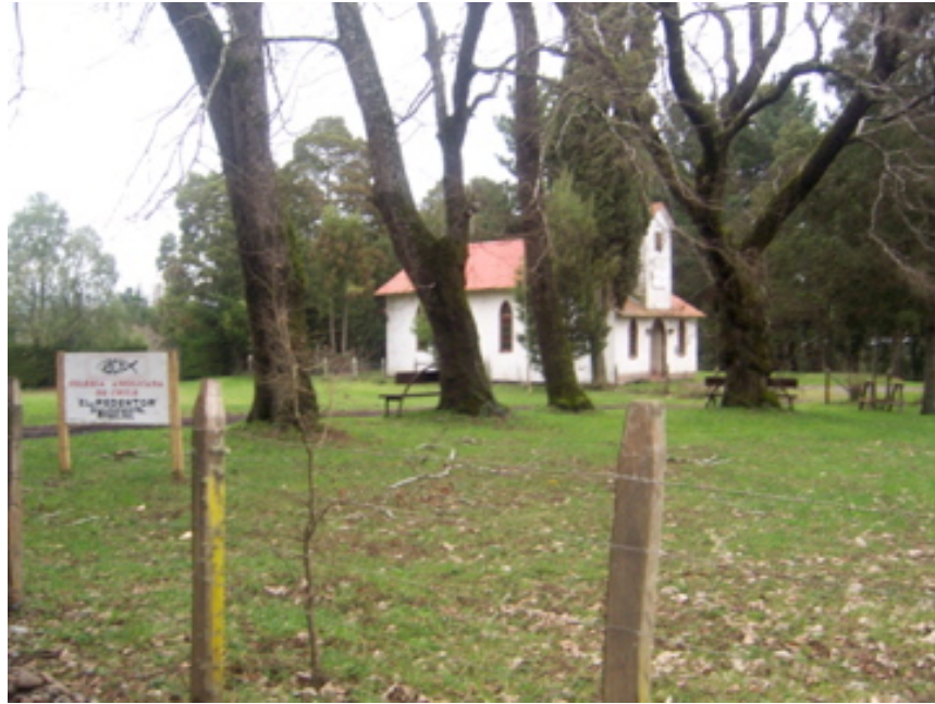
Figure 2.8: Anglican Mission Church to which Hospital Makewe formerly belonged
