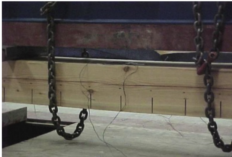
Fig. 8. Mid-span cracks details of the pre-damaged wood beam of Group "A".
