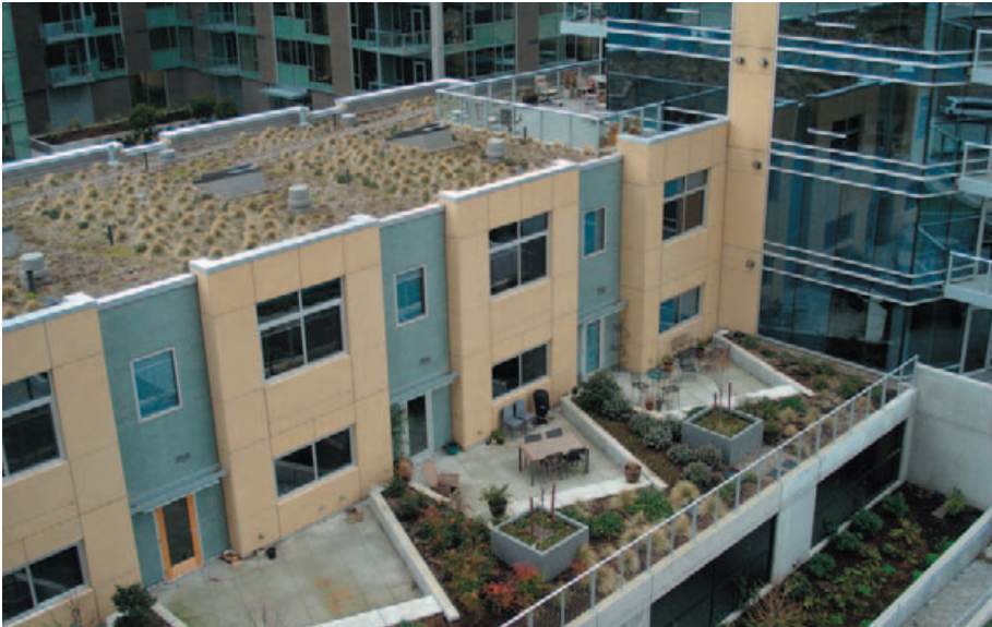
Figure 5a, New green roof at South Waterfront high-density building
