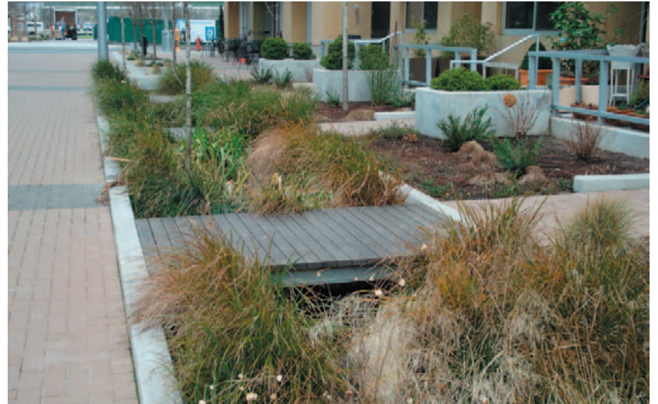
Figure 5b, Flow-through planters at South Waterfront
