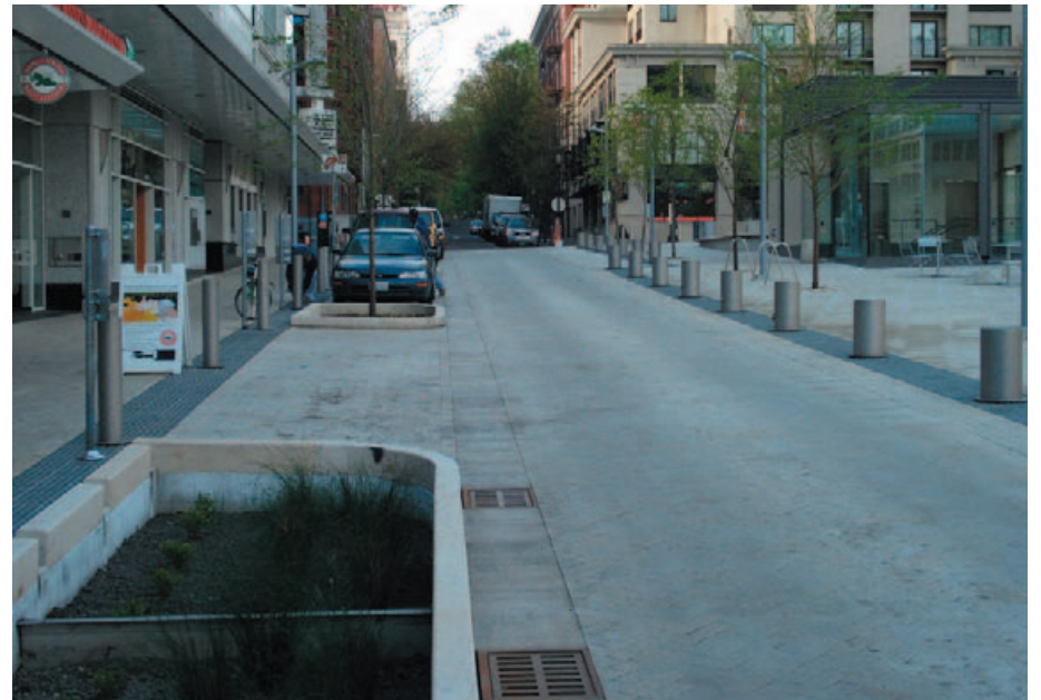
Figure 5d, Flow-through planters at new Director Park plaza street
