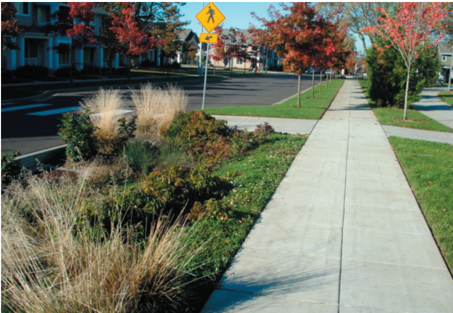
Figure 5c, Flow-through planter at New Columbia low-income neighborhood
