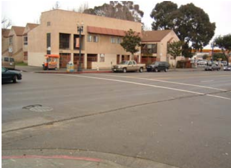
Looking southeast with view of southerly crosswalk
