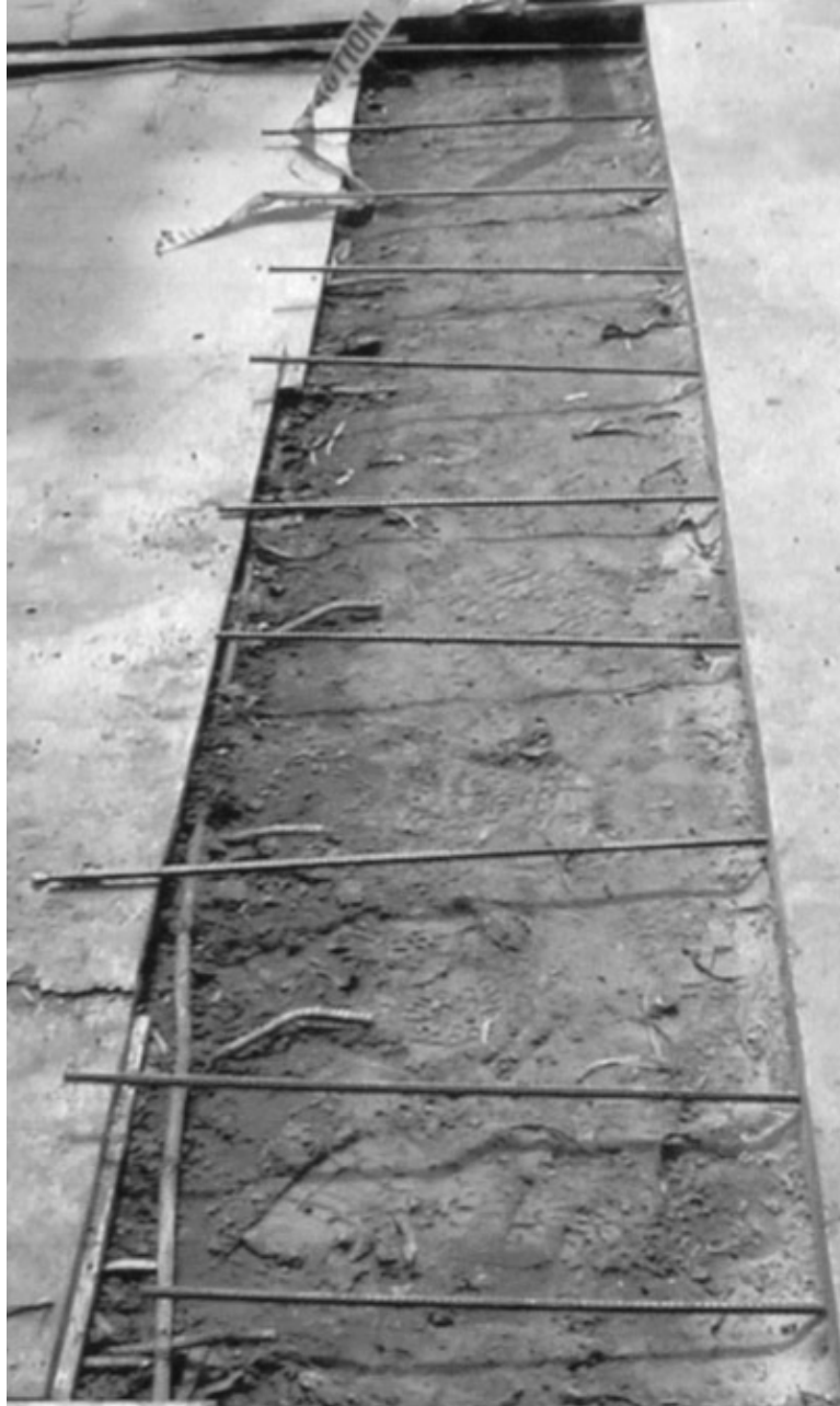
Figure 4.1: Imaged walkway area and reinforcement bars prior to concrete overlay.
