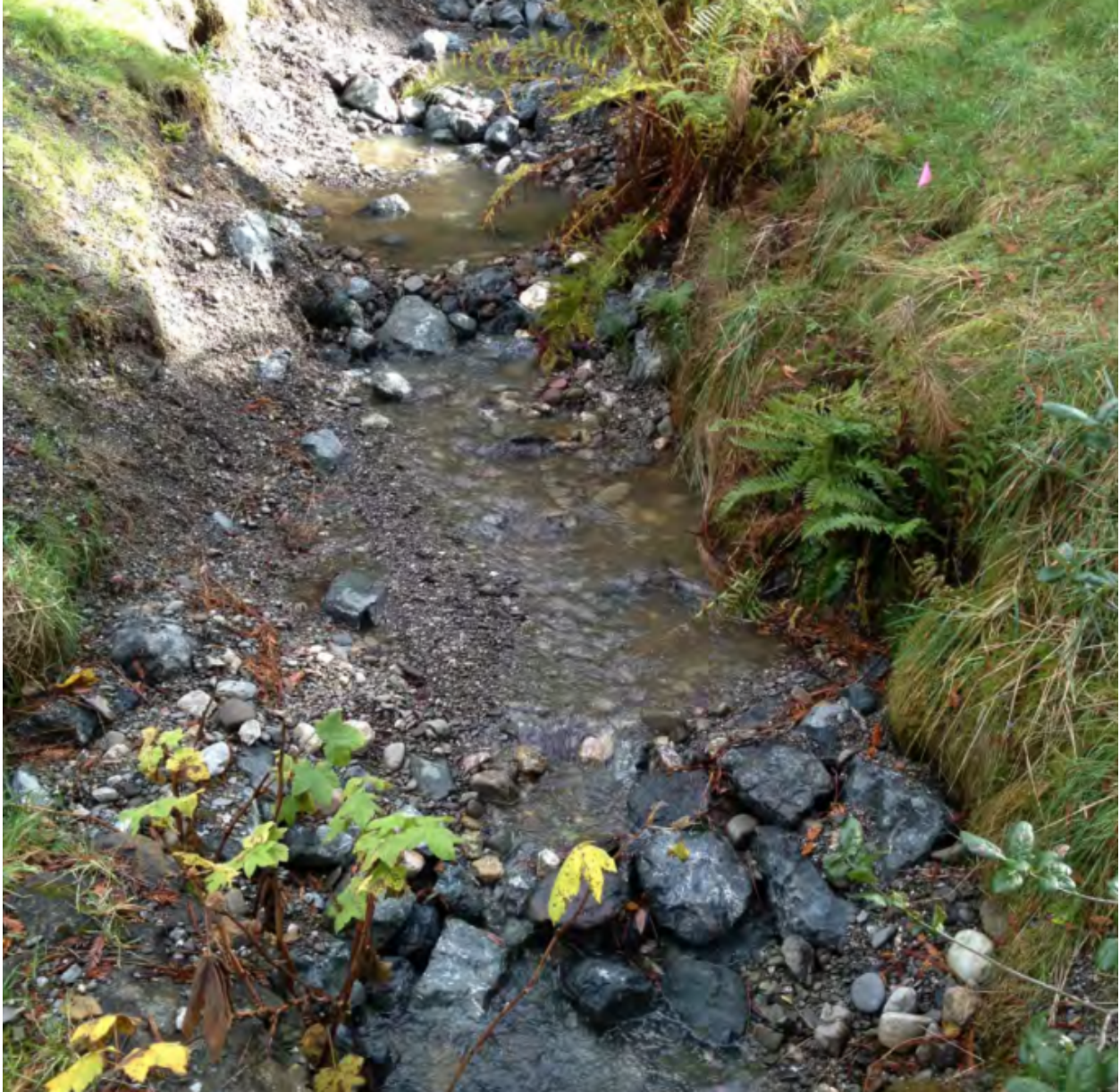
Figure 17a: Experimental Reach on Wildcat Creek, Berkeley, CA. Photo Point 7, taken immediately post-construction in 2012. The grouping of large rocks as steps and areas with smaller sediment as pools is very clear at this point in time.
