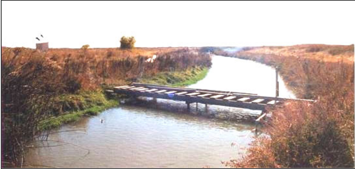
Figure 2.9. Los Baños Creek at the Highway 140 monitoring station.
