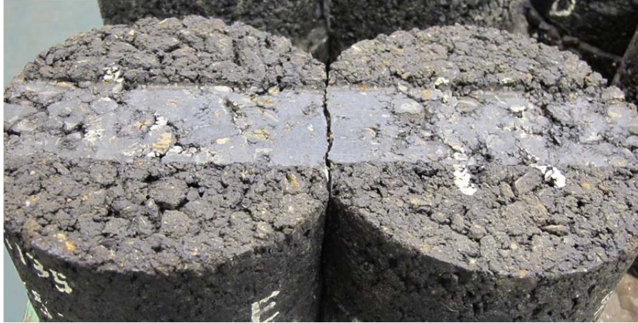
Figure 2.16: HMA cores following HWTT testing.
