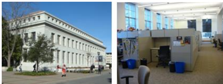
Figure 2 – Building east facade and interior cubicles
