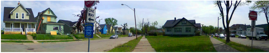
Figure 2. In the spring of 2011, a tornado in North Minneapolis damaged hundreds of homes and the large trees that lined the streets.
