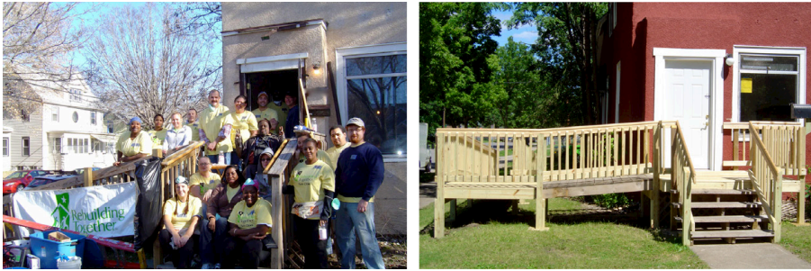
Figure 5. Accessibility ramp and exterior repairs for this low-income homeowner helped to make the home safer and more personal.
