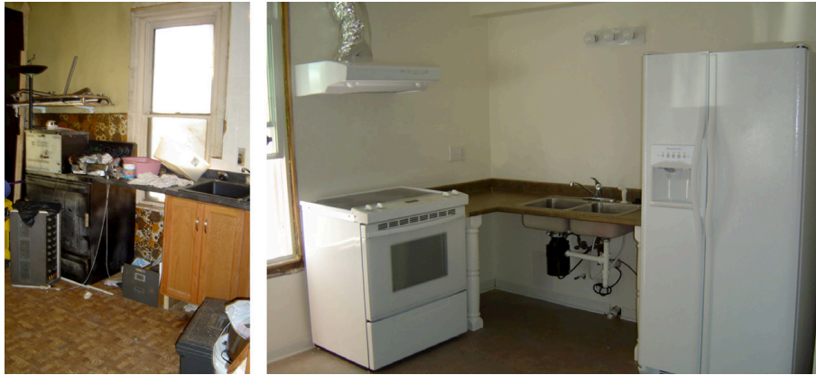
Figure 4. A kitchen renovation done by Rebuilding Together Twin Cities.
