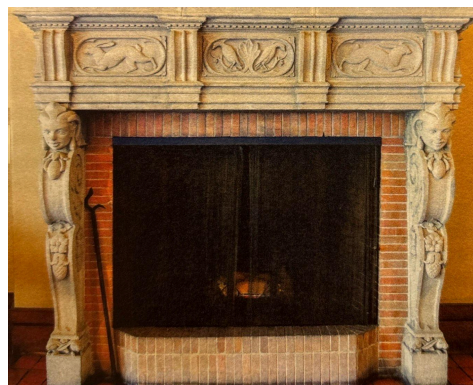
Figure 2.12 (above). Cast stone flower ornamentation on the Theater Room fireplace.
