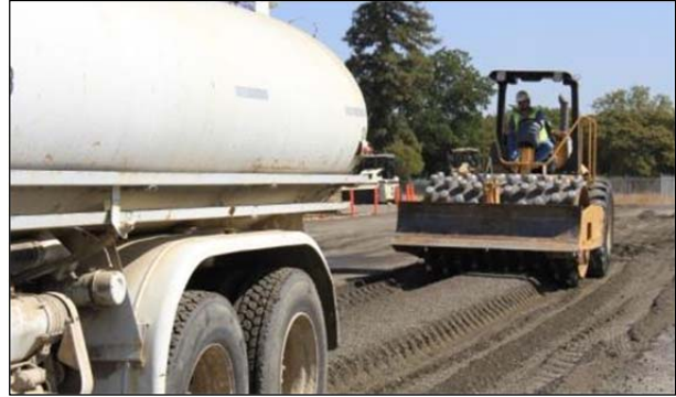
Figure 3.9: FDR-NS: Initial compaction with padfoot roller.
