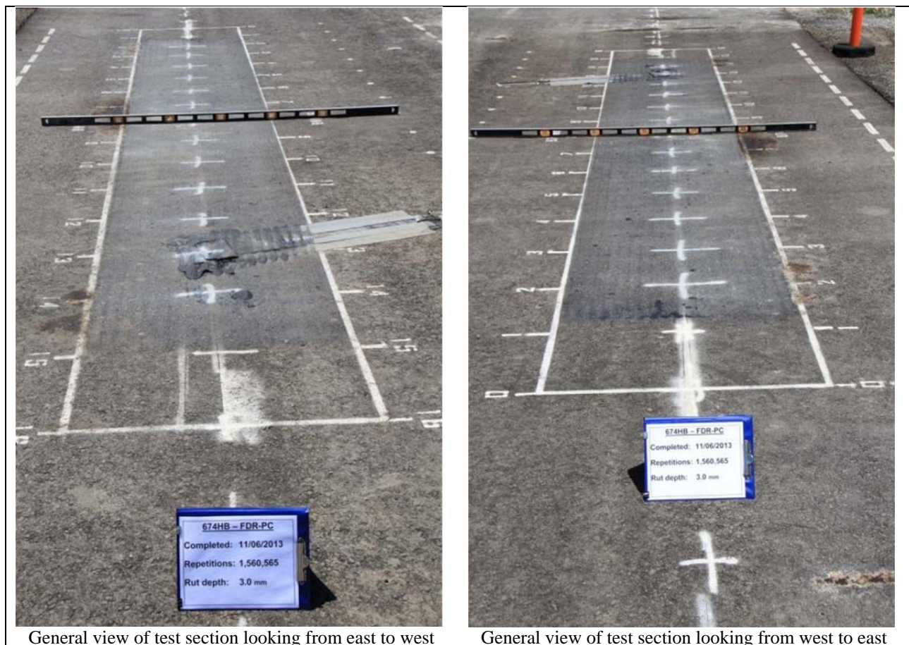
Figure 5.64: 674HB: Test section photographs.
