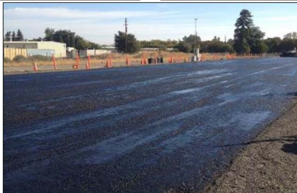
Figure 3.36: Prime coat application.
