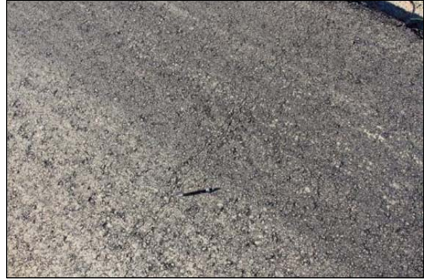
Figure 3.39: Second lift of asphalt concrete showing shearing over instrumentation cables.
