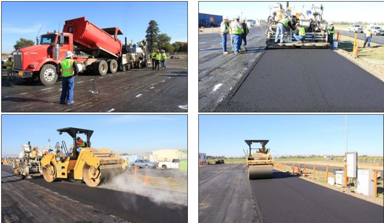
Figure 3.37: Asphalt concrete placement.
