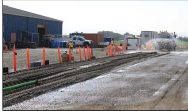
Figure 3.30: FDR-PC: Water spray prior to second mixing pass.
