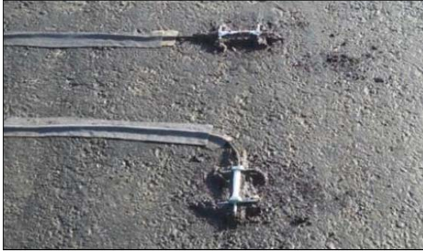
Figure 4.3: Strain gauge installation.
