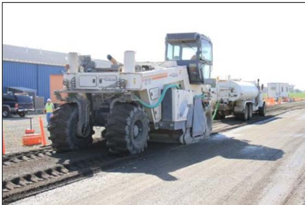
Figure 3.31: FDR-PC: Second mixing pass with water.
