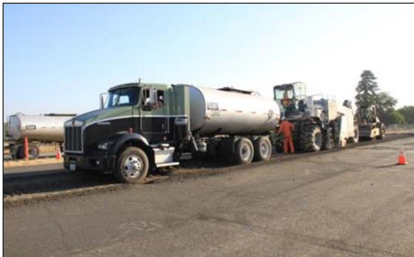
Figure 3.14: FDR-EE: Recycling train.
