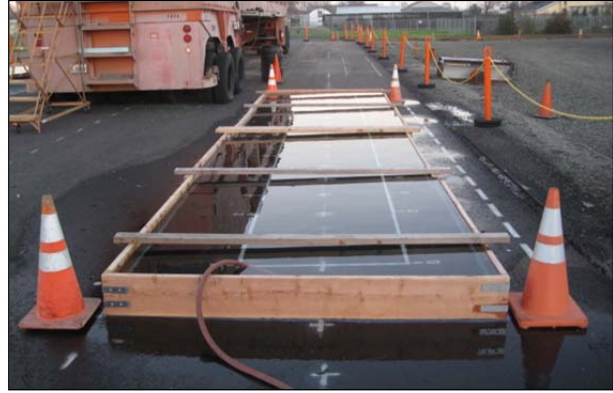
Figure 4.11: Water dam on test section.
