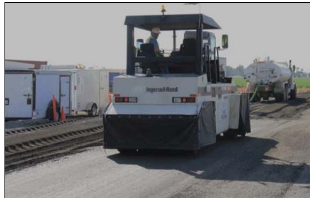
Figure 3.26: FDR-FA: Final compaction showing tightly bound surface.
