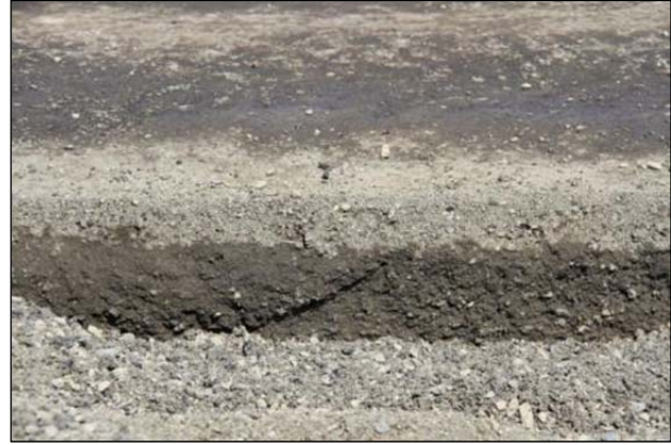
Figure 3.20: FDR-EE: Excavation showing wet recycled layer.
