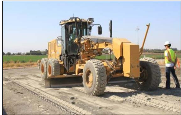
Figure 3.28: FDR-PC: Removing excess cement on Cell #8.
