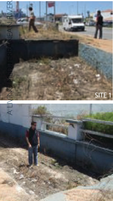
Site 1 includes an existing concrete basin between two industrial buildings which could be used to detain water as drawn in the section illustration (right).
