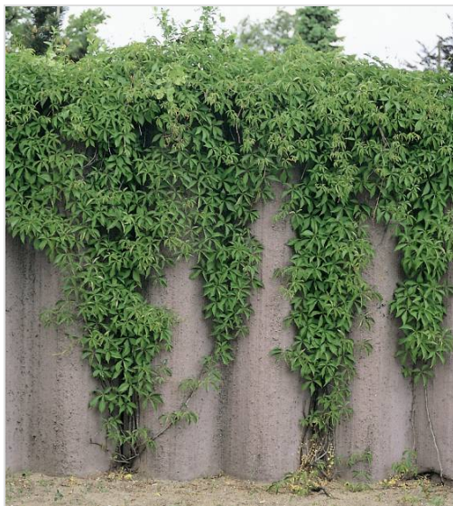
Figure 3.25. Colored concrete noise barrier made of 8 cm (3 in.) thick corrugated element with green vegetation at National Road 405 in Århus, Denmark [1, 3].
