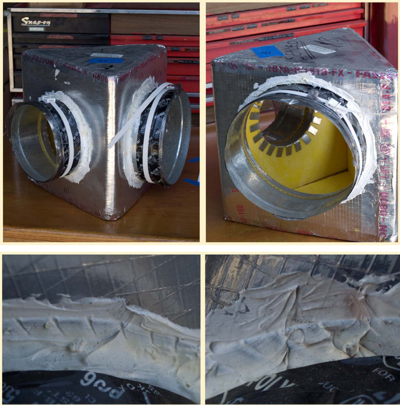
Figure 19. Splitter box starter collars sealed with mastic.
