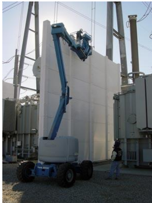
Figure 108 Composites fabricated from Wo-PCs, a) firewalls made of PCs composite panels reinforced with fibers for protection of electric transformers, b) detail of the panels installation.
