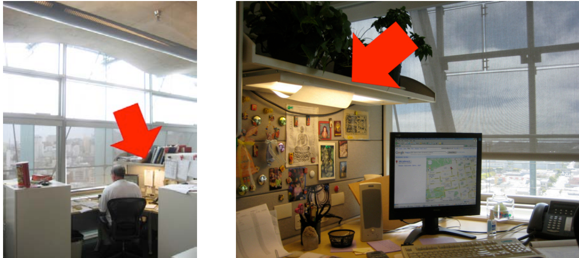
Figure 10.9 Location of task lighting installed in workspace partitions on NW (left) and SE (right) perimeter zones. Note occupant intervention for glare control in righthand image.
