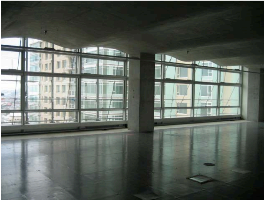
Figure 11.1 Interior view of the SE perimeter zone prior to occupancy showing floor to ceiling high VLT glass window wall typical for both NW and SE facades.
