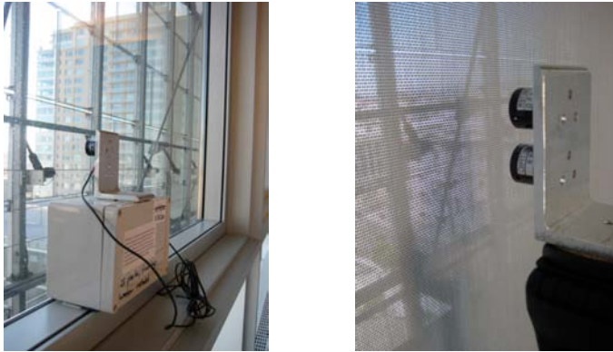
Figure 4.10 Vertical (unshaded) irradiance at glass (left) and vertical (shaded) irradiance and illuminance at 2” from interior face of roller shade fabric (right).
