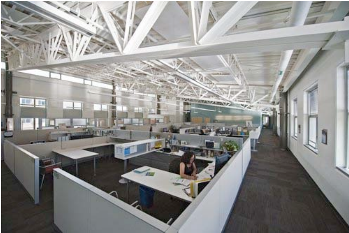
Figure 11.16 Lightlouver™ OLS installed in National Renewable Energy Laboratory (NREL) Research Support Facility (RSF).
