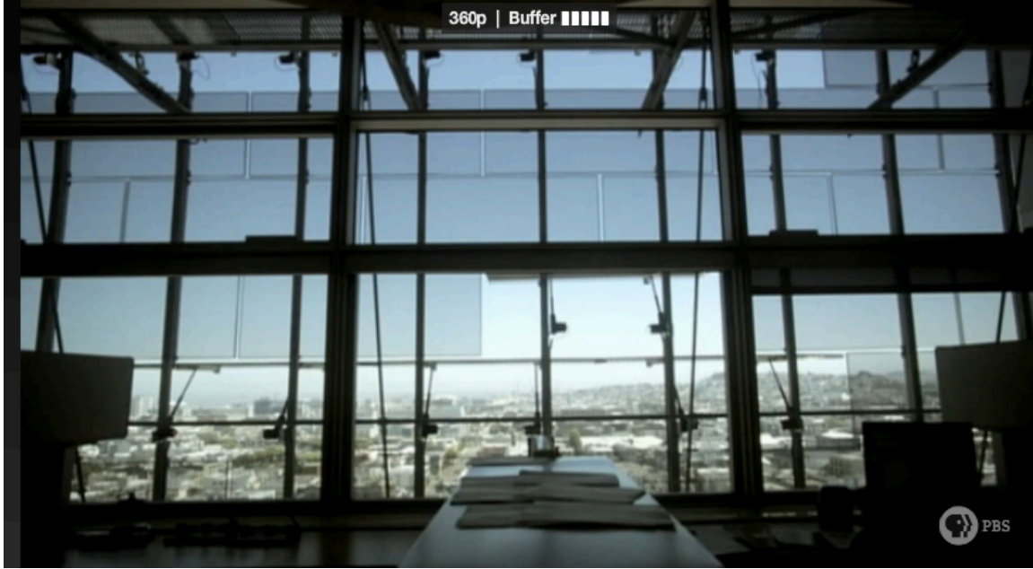
Figure 3.10 Interior view looking through SE facade at exterior metal screen. Image shows select panels that are open. From PBS Design e2 podcast entitled “Greening the Federal Government.” 13
