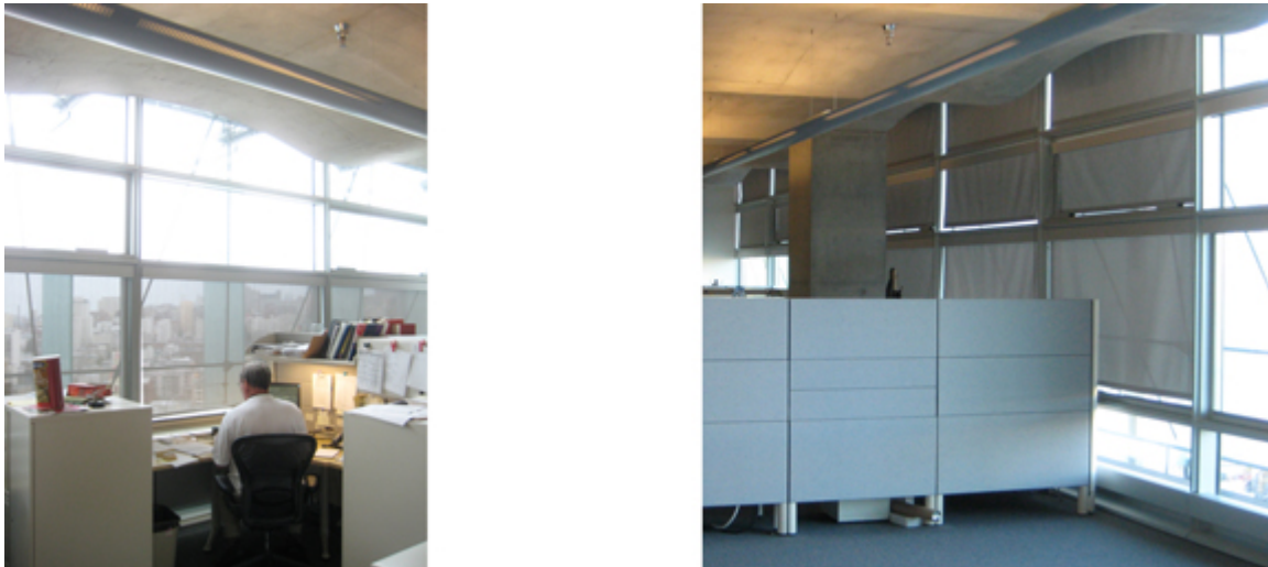
Figure 5.2 Overview of NW facade workstations where interior roller shades were added to the row of vision windows only (left) and to the upper two rows of windows in addition to the vision windows (right). The openness factor for shades in both images is the same (5%). The difference in perceived transparency is the result of different camera exposure settings.
