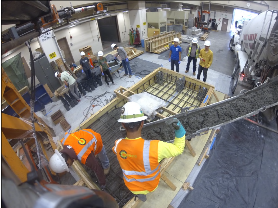
Figure G- 20. Specimen casting November 21, 2017
