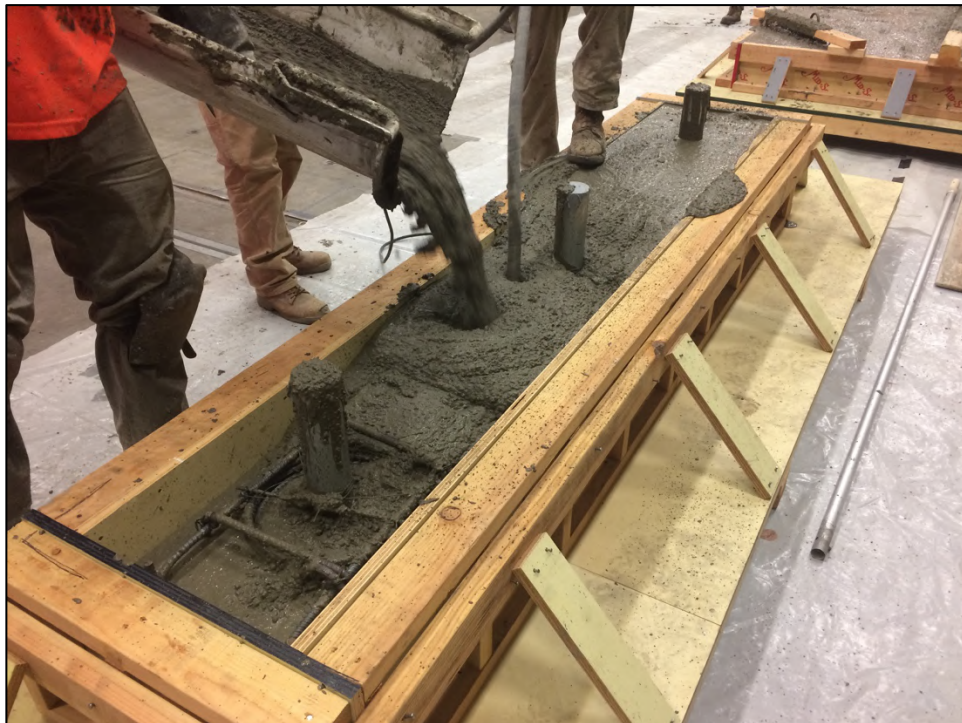
Figure G- 10. Support type 2 casting October 25, 2017
