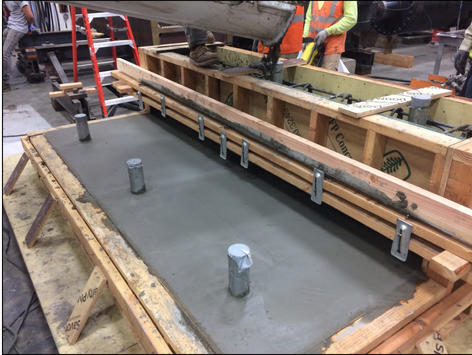
Figure G- 9. Support type 1 casting top section October 25, 2017 #2
