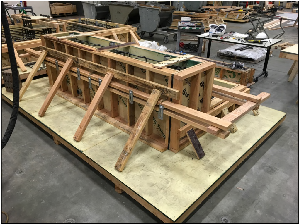
Figure G- 4. Support type 1 form with reinforcement ready to cast #2
