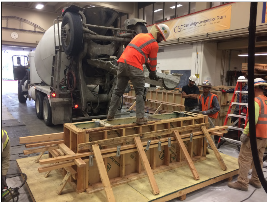
Figure G- 8. Support type 1 casting top section October 25, 2017 #1
