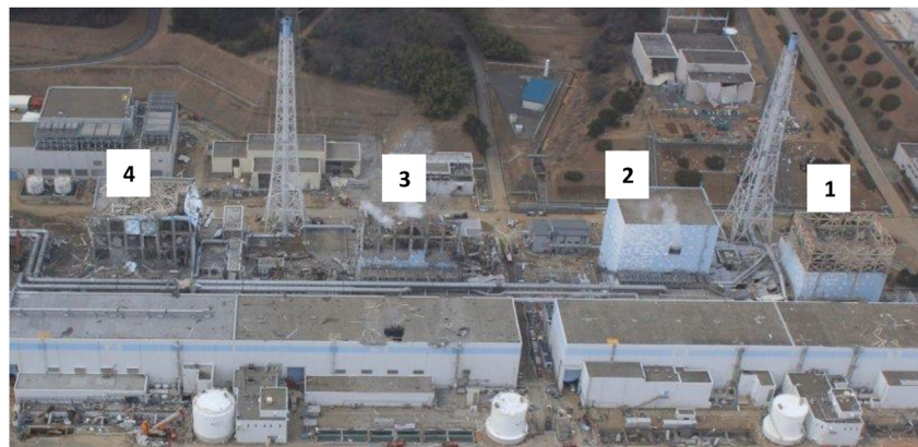
Figure 3. The status of the FDNPP Units 1, 2, 3, and 4 after the accident (retrieved and modified from the American Nuclear Society schematic, https://www.ans.org/news/article-2672/fukushima-daiichi-10-years-on/ )
