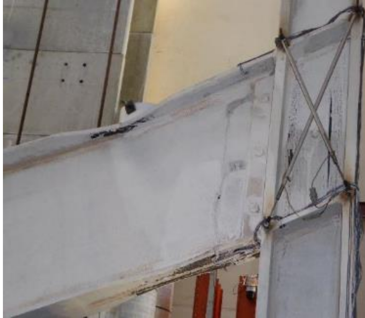
(a) View from East
