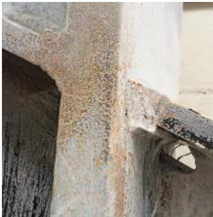
(b) Detail A, Top Flange CJP Weld
