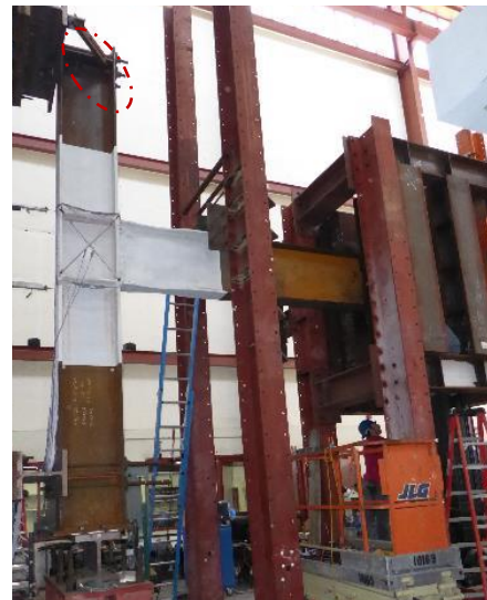
(c) View from West
