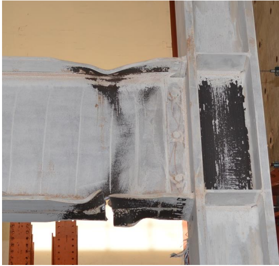
(a) View from East
