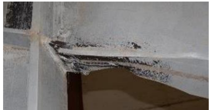
(c) View of Beam Bottom Flange
