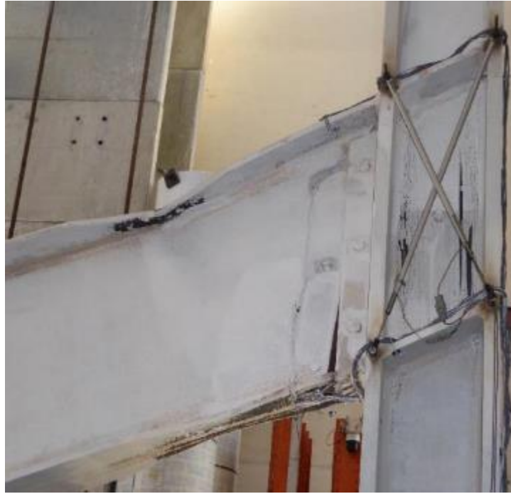
(a) View from East
