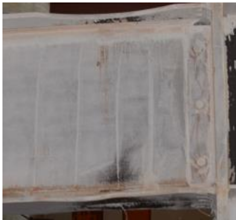
(e) Detail C, Minor Flange and Web Local Buckling
