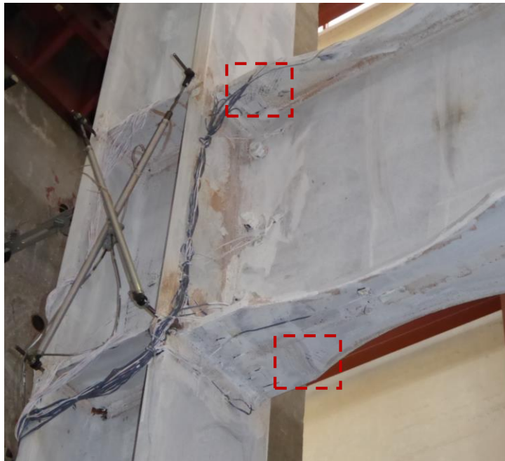
Figure 3.31 Specimen C2 Beam Flange Yielding at Completion of 0.01 rad Drift Cycles
