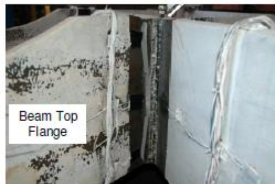
(b) Close-up View of The Fracture
