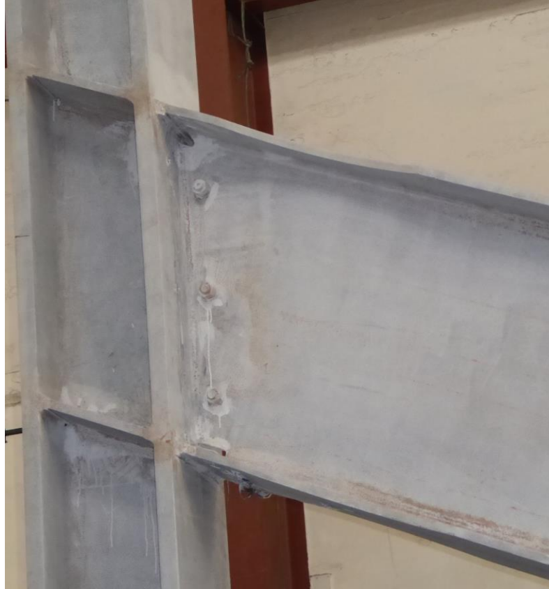
Figure 5.20 Specimen S1 Connection Prior to Testing
