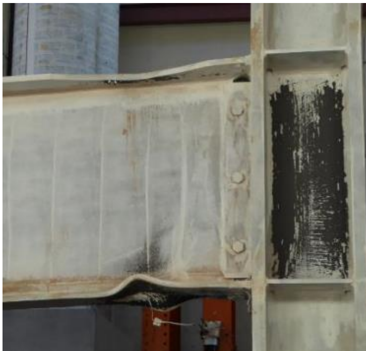
(a) View from East
